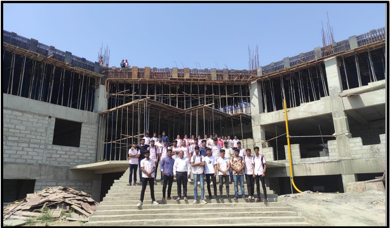
Fig.3: Students at construction site of AI COE building.
