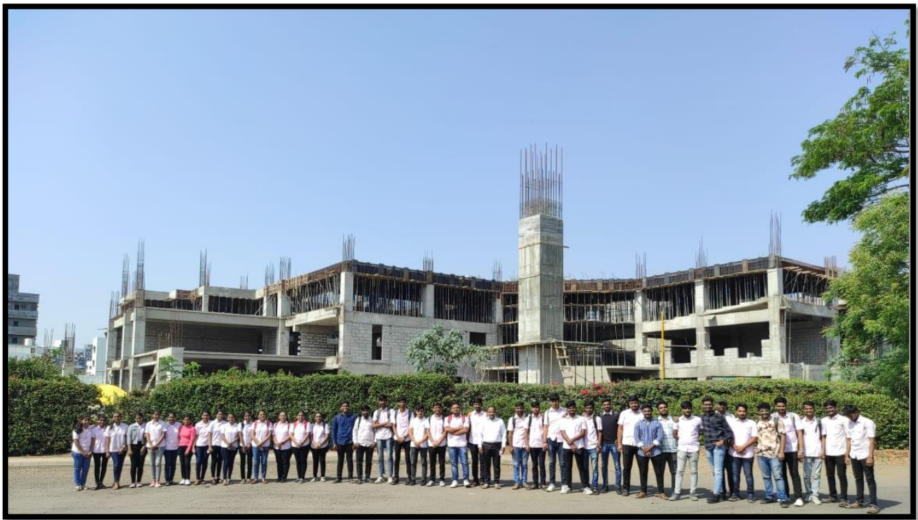
Fig 1: students in Campus near Boys hostel and CBSE school, Playground (AI COE building construction site in background)
